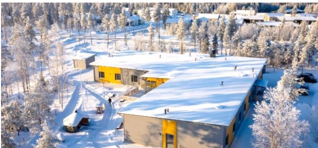
Kempele Ihmemaantie in Kempele (FI) Development project completed on 22 January 2021
