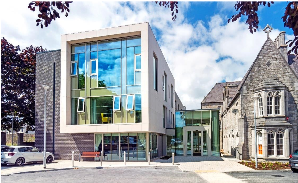
Clondalkin Nursing Home in Clondalkin (IE) Care home completed in July 2023
