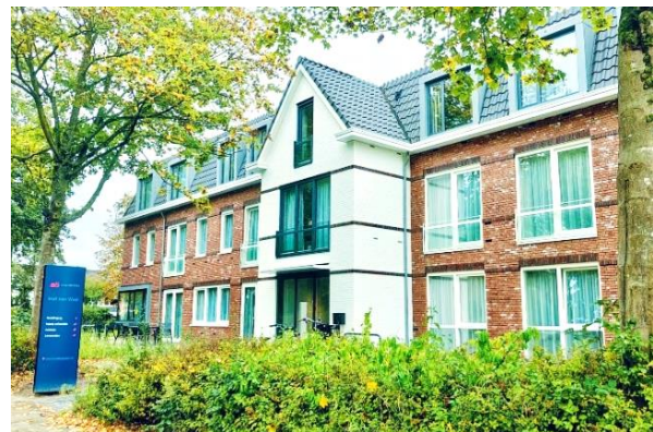
Hof van Waal in Tiel (NL) Care residence completed in July 2023
