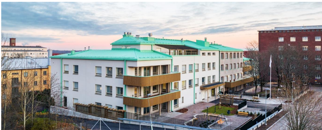
Helsinki Ensikodintie in Helsinki (FI) Shelter completed in November 2023
