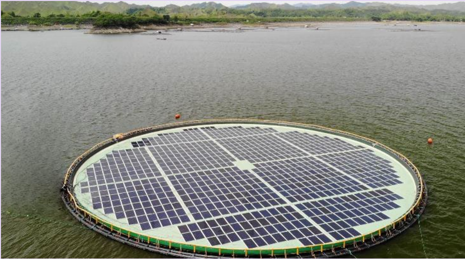
SN Power Phillipines: OceanSun Pilot on Magat dam
