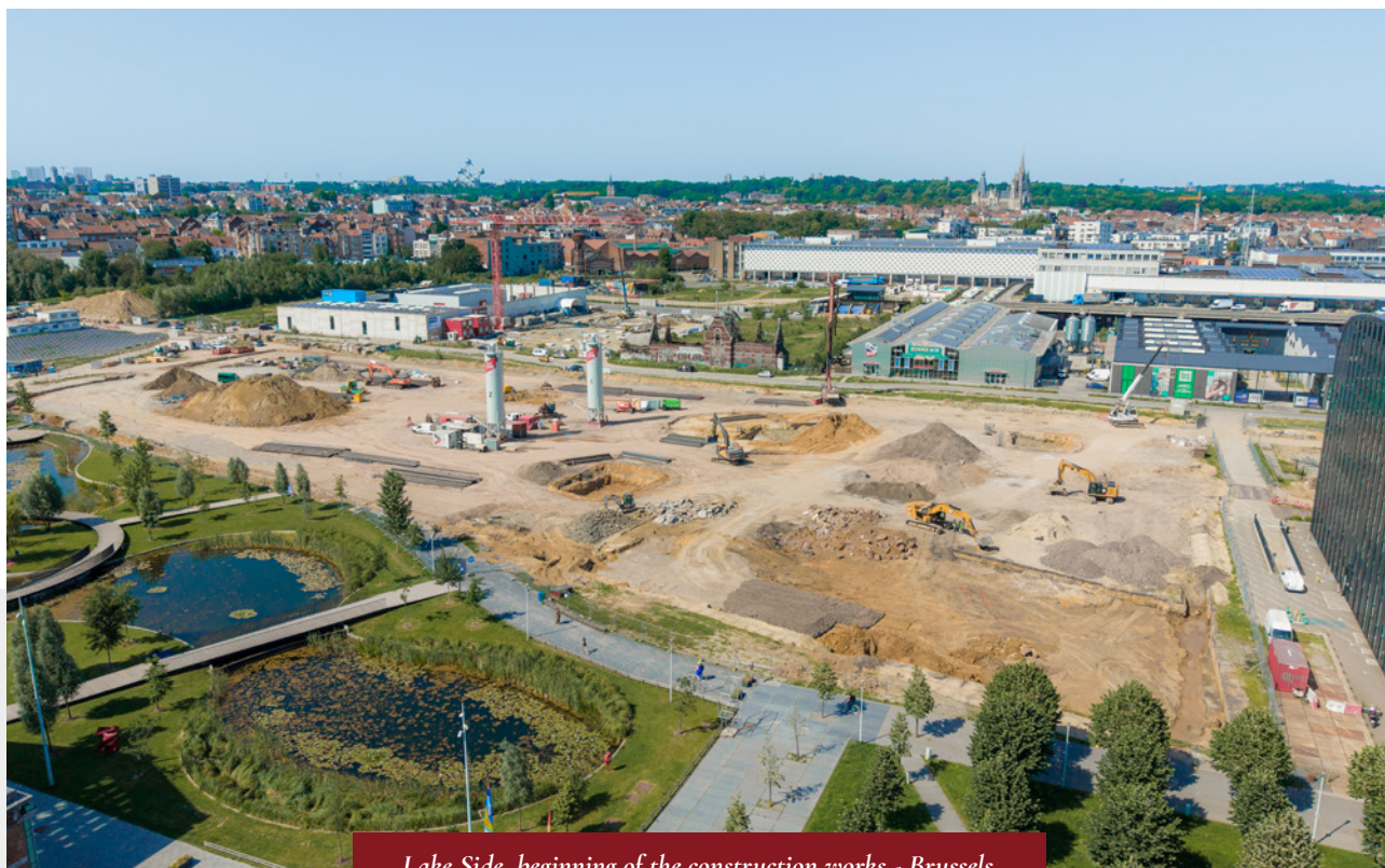
Lake Side, beginning of the construction works - Brussels
