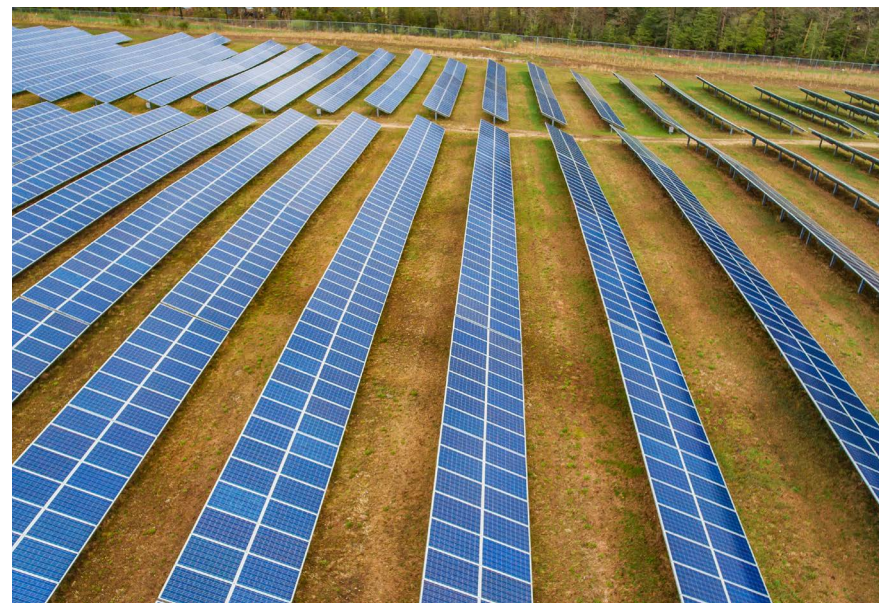
Oak solar farm in New Jersey, US is comprised of 53,200 fixed solar panels and has a capacity of 10MW.
