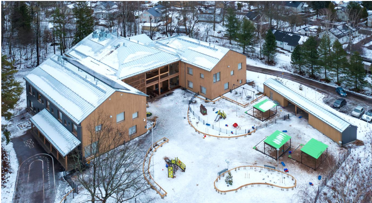
Helsinki Käräjätuvantie in Helsinki (FI) Childcare centre completed in December 2024
