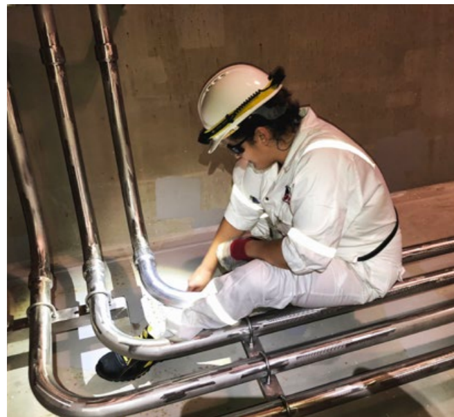
Drydocking Superintendent Yoana Leon Valdivia inspecting a tank onboard Bow Triumph.
