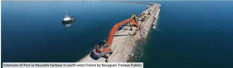
Extension of Port-la-Nouvelle harbour in south-west France by Bouygues Travaux Publics
