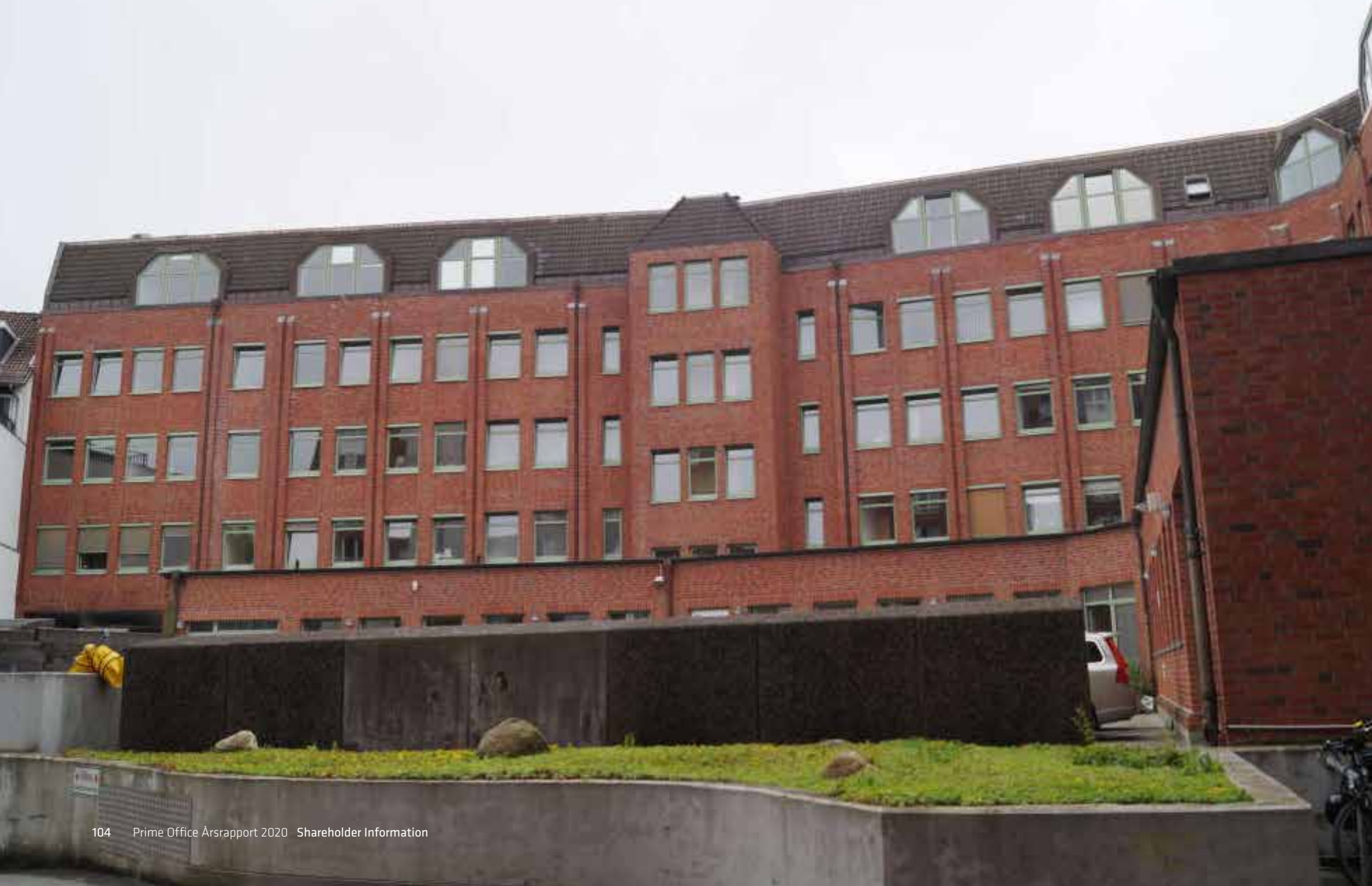
Walkerdamm i Kiel, bagside.
