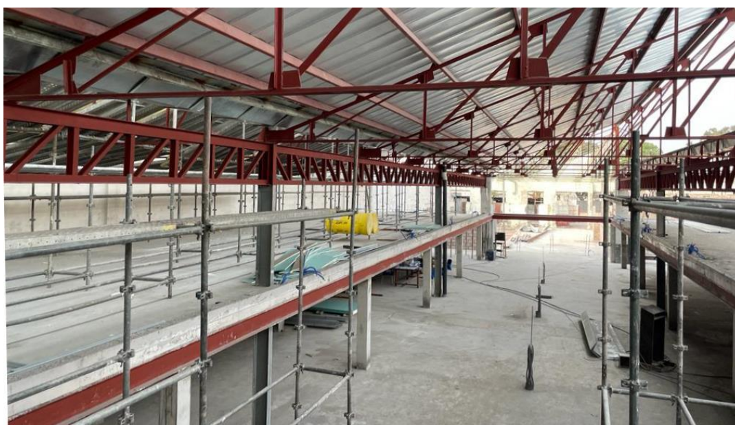
Construction site Silikin Village Phase III
