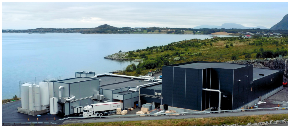
Midsund facility after 2020 build-out
