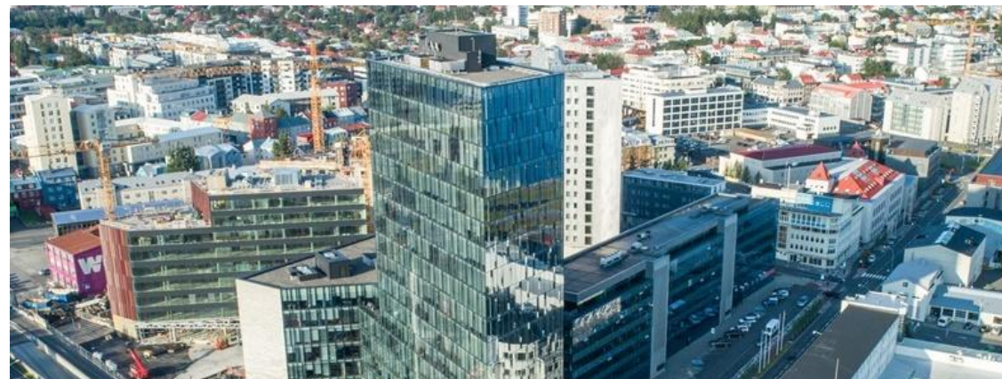
Höfðatorg Offices – 37,867 m 2
