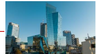
Artery Business Centre Completed in 2023
