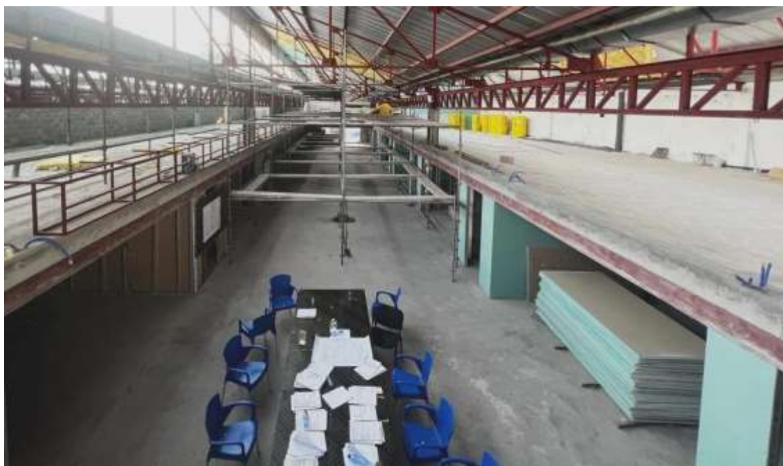
Construction site Silikin Village III
