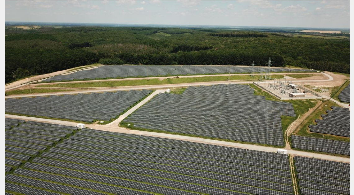
The 54 MW Boguslav solar plant in Ukraine.
