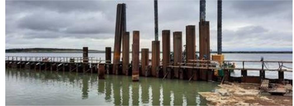
**RECONSTRUCTION OF BERTHS. PHASE I. CONSTRUCTION OF NEW BERTH. INSTALLATION OF THE SUPRASTRUCTURE** Construction works are underway, installation of berth load-bearing structures and engineering networks, technological pipelines
