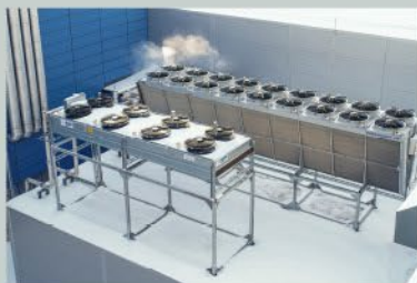
Picture of the cooling towers of the new process water cooler and recycler
