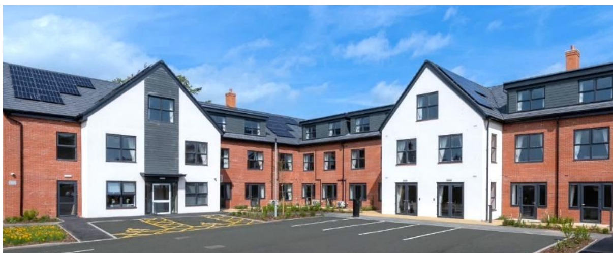
Beechwood Care Centre – Bridlington Care home acquired in July 2026
