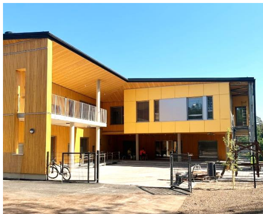
Espoo Kuurinkallio in Espoo (FI) Service community completed in May 2024
