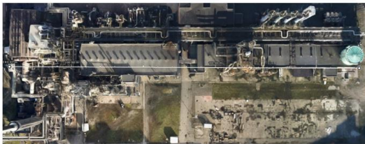
Comparison of footprint: Hilli Episeyo and land based Ammonia Production Facility of similar production volume
