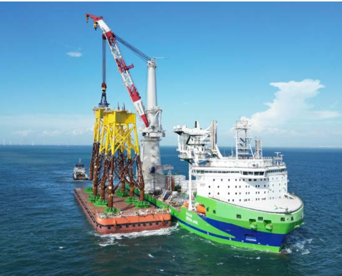
DEME • Offshore Energy, Zhong Neng
