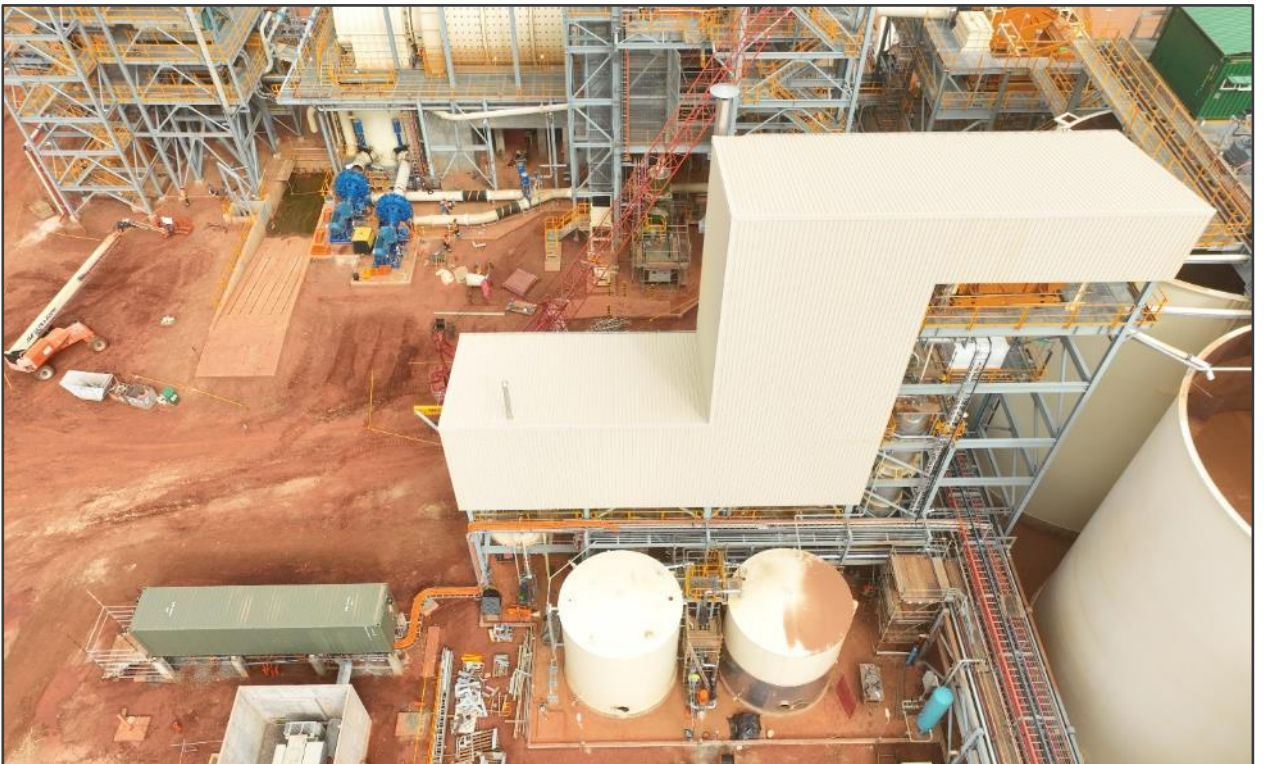
Figure 6: Completed elution circuit
