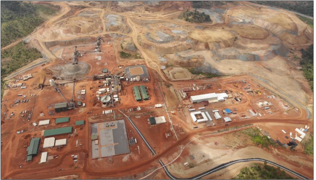
Figure 1: Lafigué processing plant overview with project construction 94% complete
