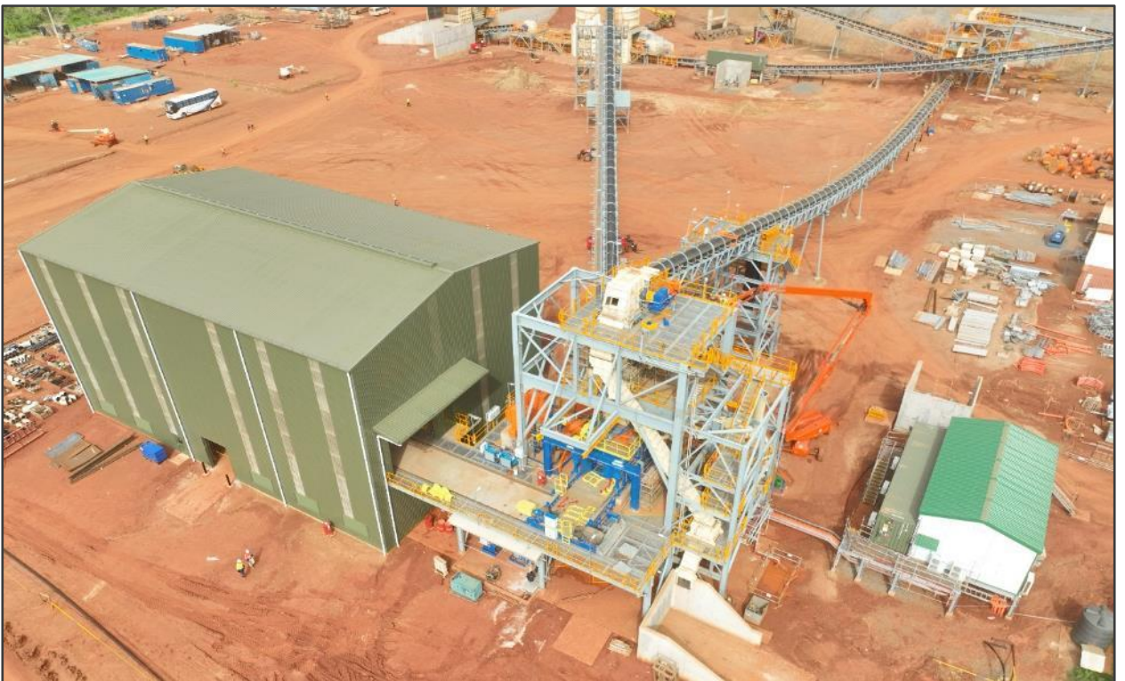
Figure 4: Wet commissioning of HPGR is underway
