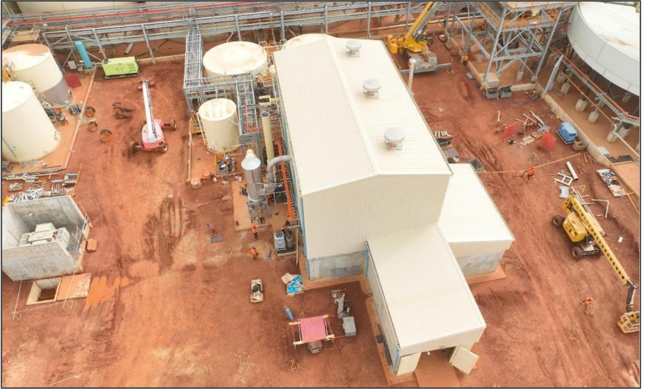
Figure 7: Gold room construction is now largely complete
