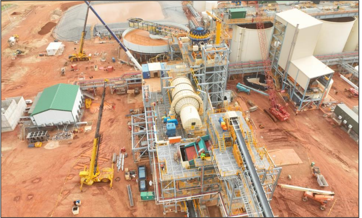
Figure 3: Wet commissioning of the ball mill is underway
