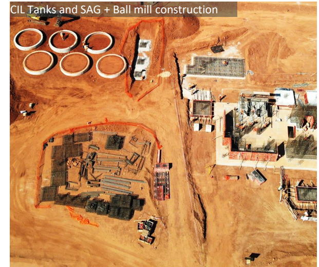
CIL Tanks and SAG + Ball mill construction
