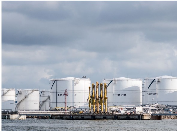
LIQUID ENERGY terminals
