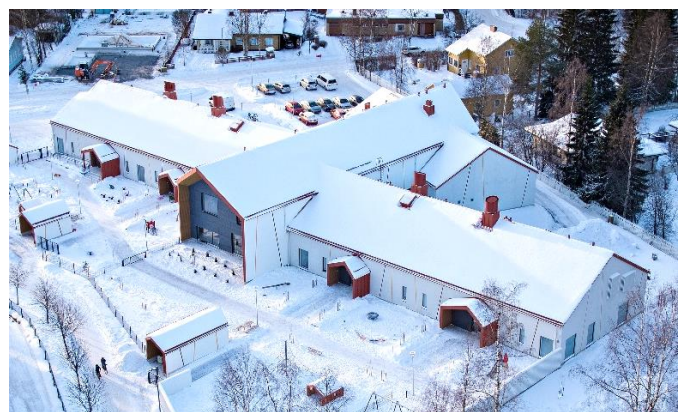
Oulu Valjastie in Oulu (FI) Development project completed in November 2021
