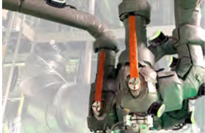
*The NIBE subsidiary BriskHeat produces high-performing, energy-efficient heating jackets with temperature control. These are installed on various kinds of gas pipelines to prevent condensation and keep processes running smoothly. BriskHeat's heating jackets with control systems control and monitor each heater in the system individually for optimal energy and system performance. The result is an overall improvement in performance through the temperature control system.*
