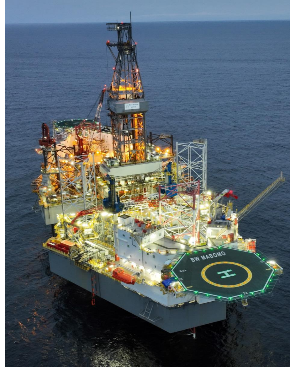
MaBoMo and Borr Norve on site in Gabon
