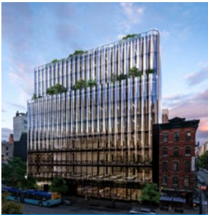
PARK VIEW (118,10TH AVE), NEW YORK, OFFICE
