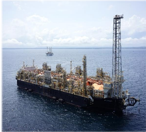
FLNG Hilli (operational) - MKI (2.4mtpa 1 )
