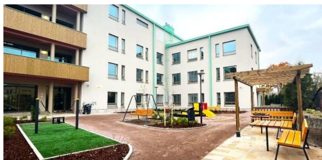
Helsinki Ensikodintie in Helsinki (FI) Shelter completed in October 2023
