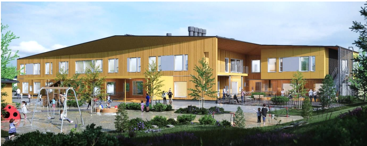
Espoo Kuurinkallio – Espoo (FI) Service community to be completed by Q2 2024
