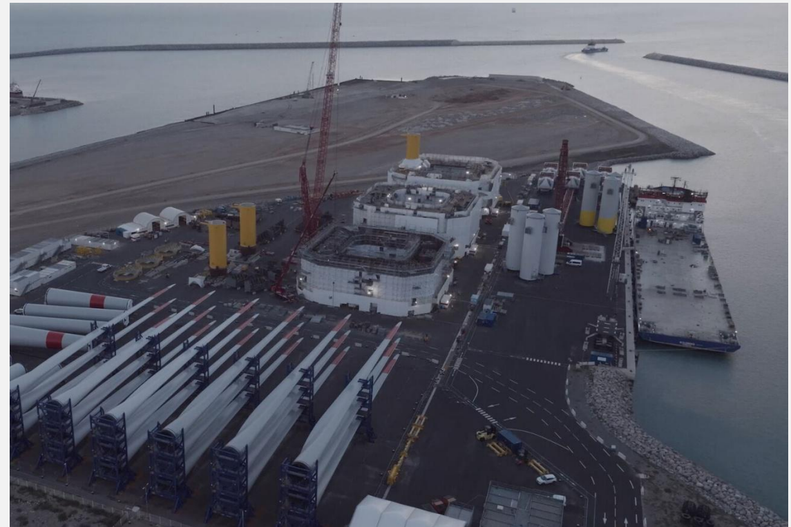
Eolmed: Assembly underway at the yard
