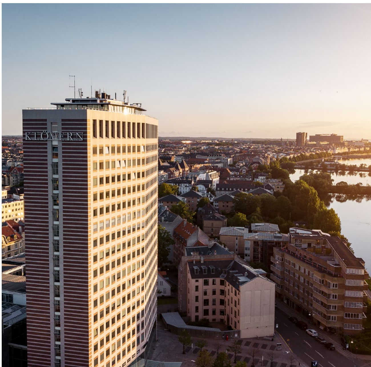
The Codan House, Copenhagen
