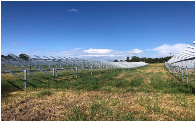
PV Energy Projects, Zaganiec construction site
