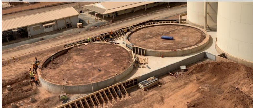
Package 4: Additional leach tank concrete base
