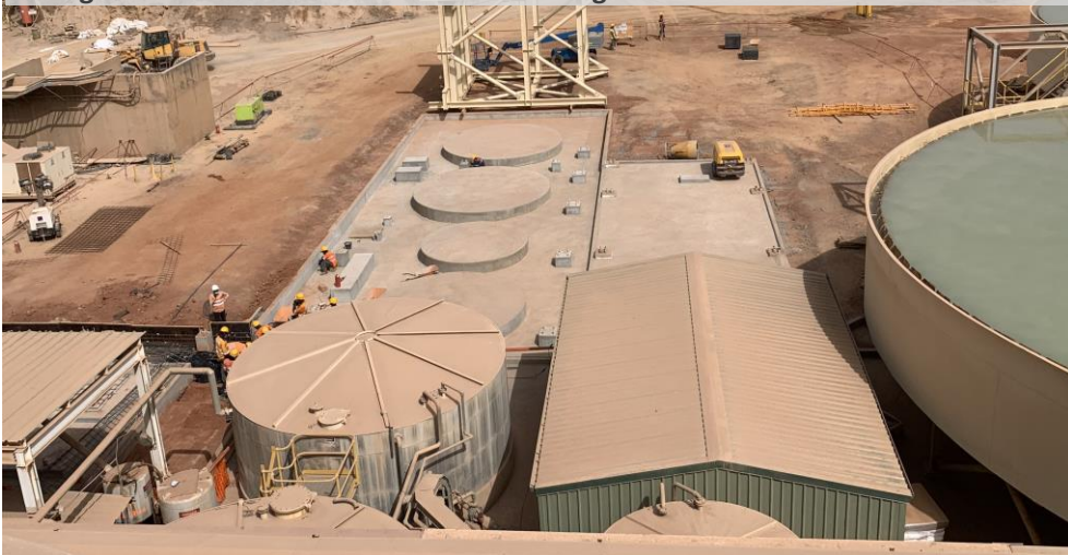
Package 2/3: Acid wash and elution columns and carbon regeneration kiln
