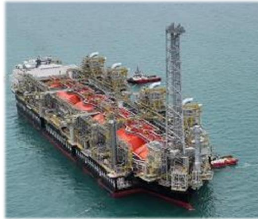
FLNG Gimi (ready for operations) – MKI (2.7mtpa)
