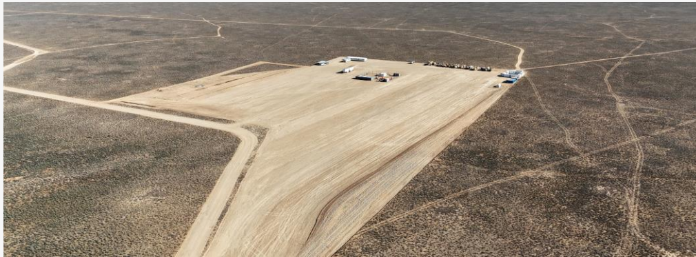
Grootfontein, South Africa, 273 MW solar
