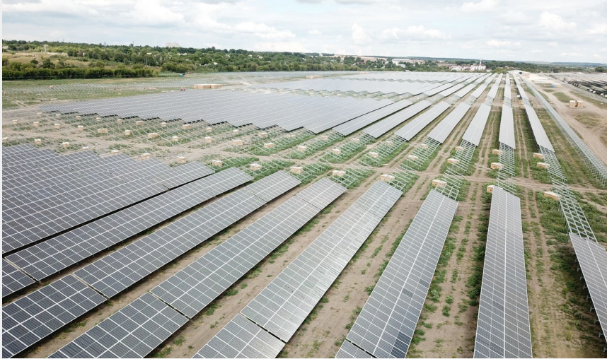
The Kamianka project under construction.
