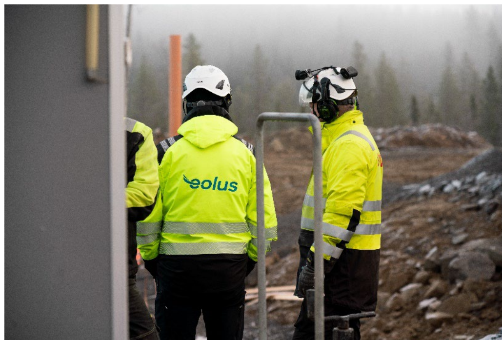
Casting of foundations for project Rosenskog, autumn 2022
