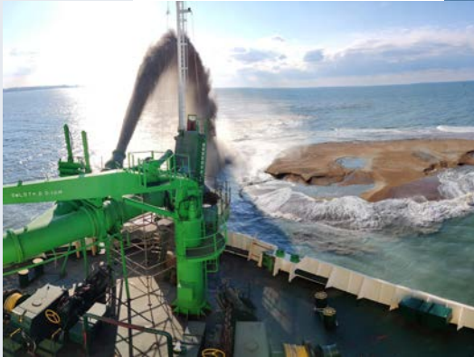
DEME > Dredging works in the Middle East
