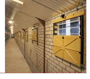
TPI Polytechniek OmniFlux' air inlet valves installed at a Dutch poultry farm
