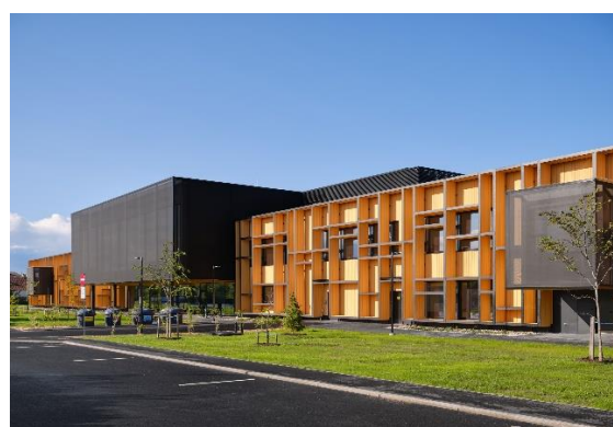
Saaremaa Upper Secondary School (Nordecon AS)
