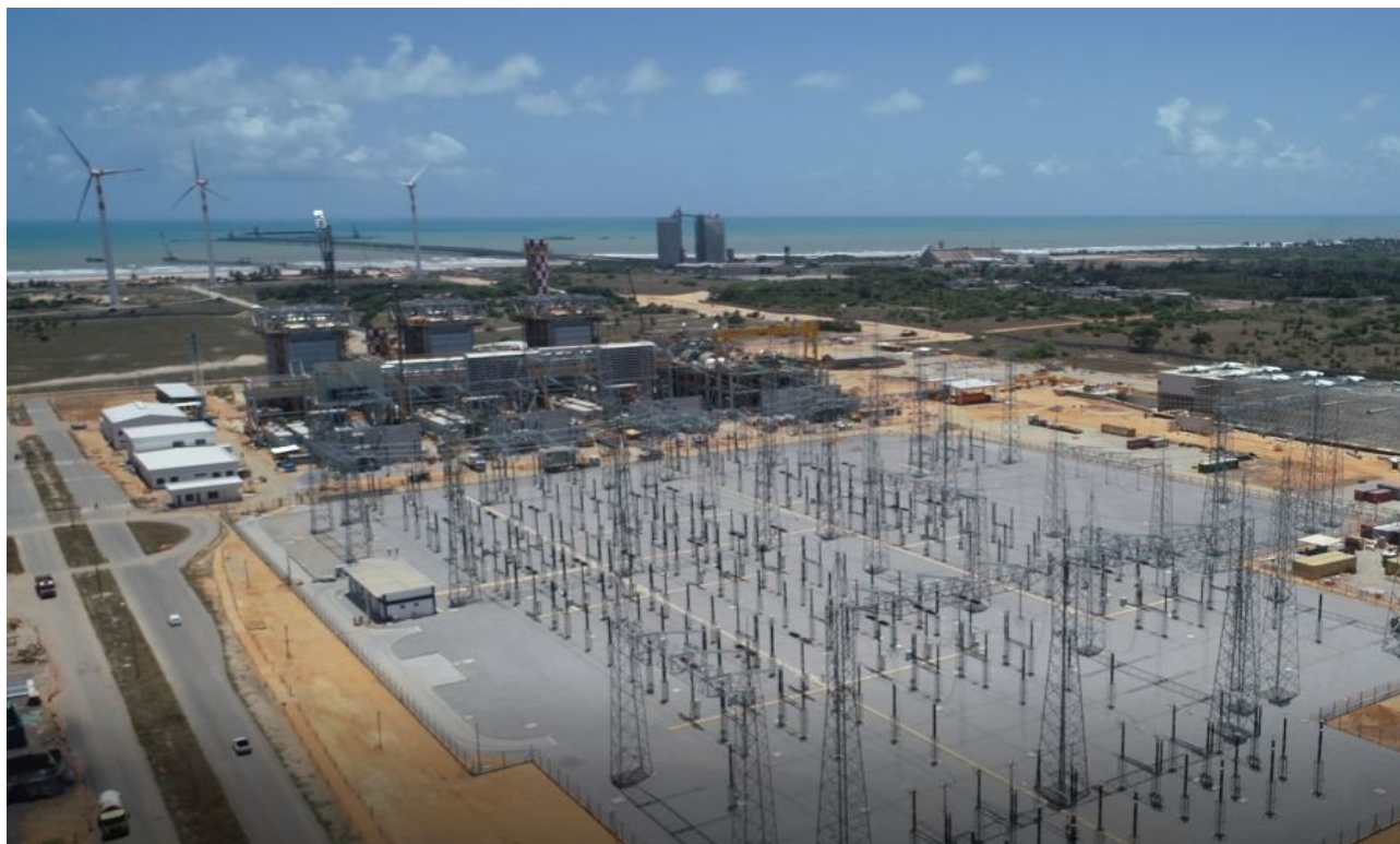
Sergipe Power Plant
