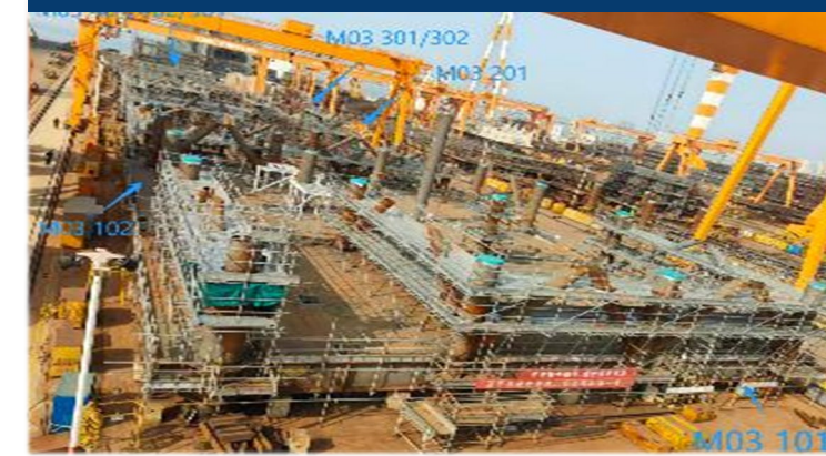
Module structural assembly ongoing
