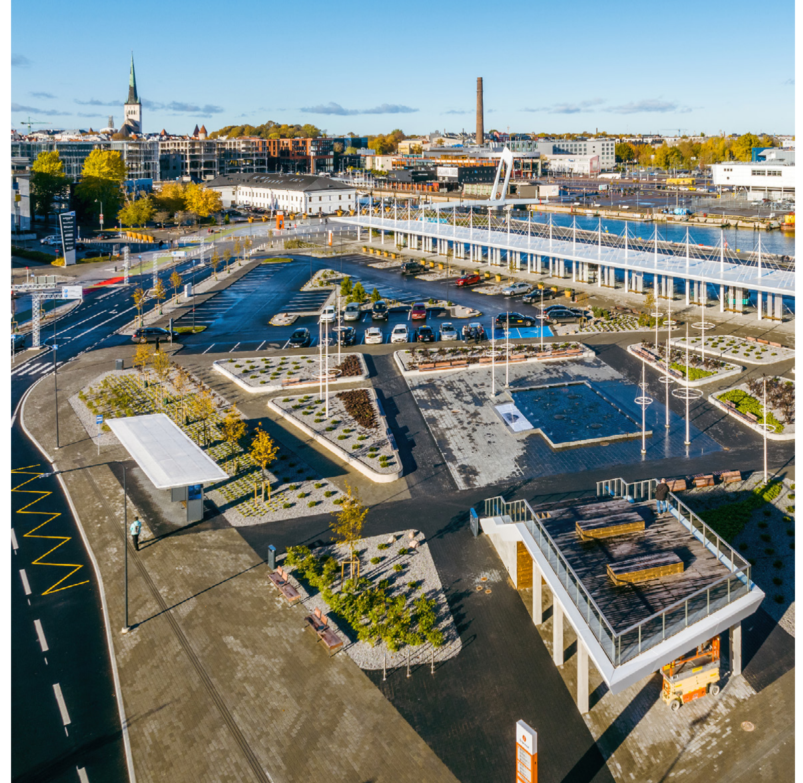
THE SQUARE IN FRONT OF PASSENGER TERMINAL D WAS COMPLETED
