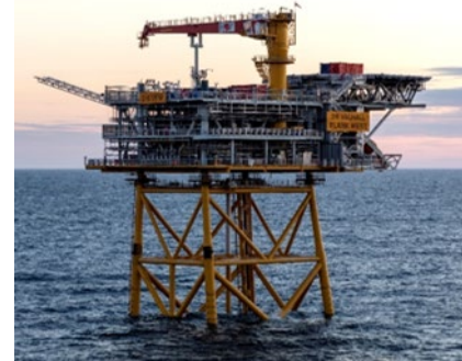
Valhall Flank West normally unmanned WHP
