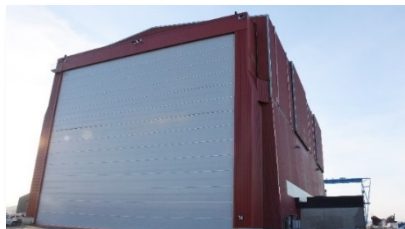
Fabrication hall, Verdal Yard
