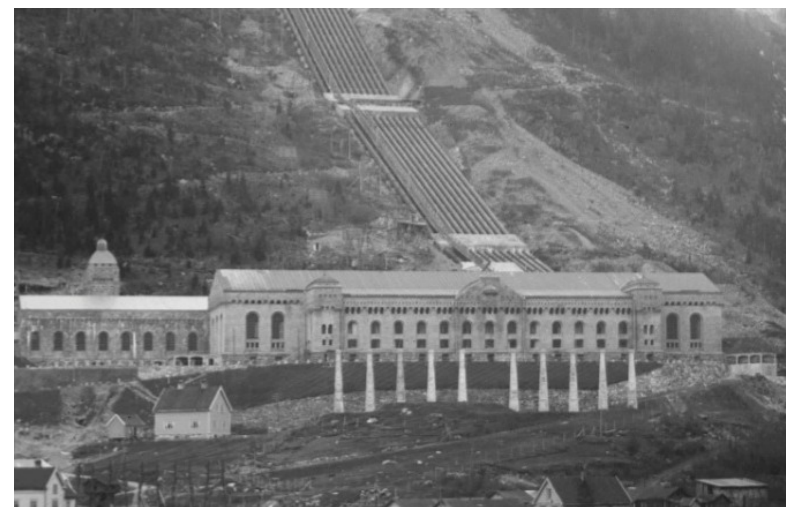
Vemork power plant: located in Rjukan, Telemark and operational since 1911
