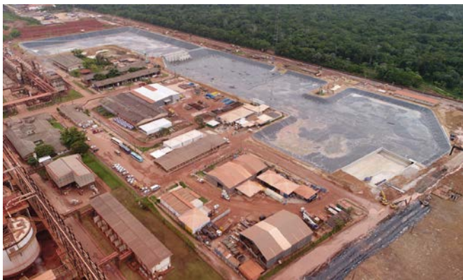
The water reservoir capacity at Alunorte has been increased by 350 percent since the rainfall event.
