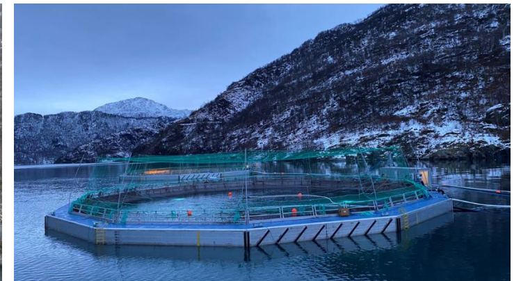
Semi-Closed Containment Systems
