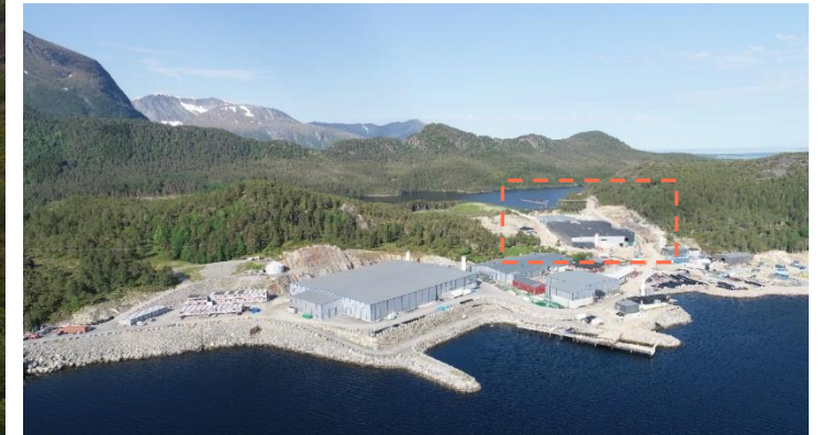
Nordheim under commissioning
