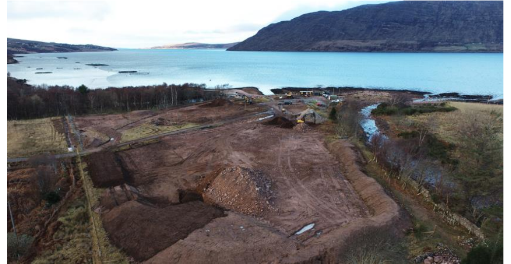
Ardessie, Scotland. Groundwork has commenced
