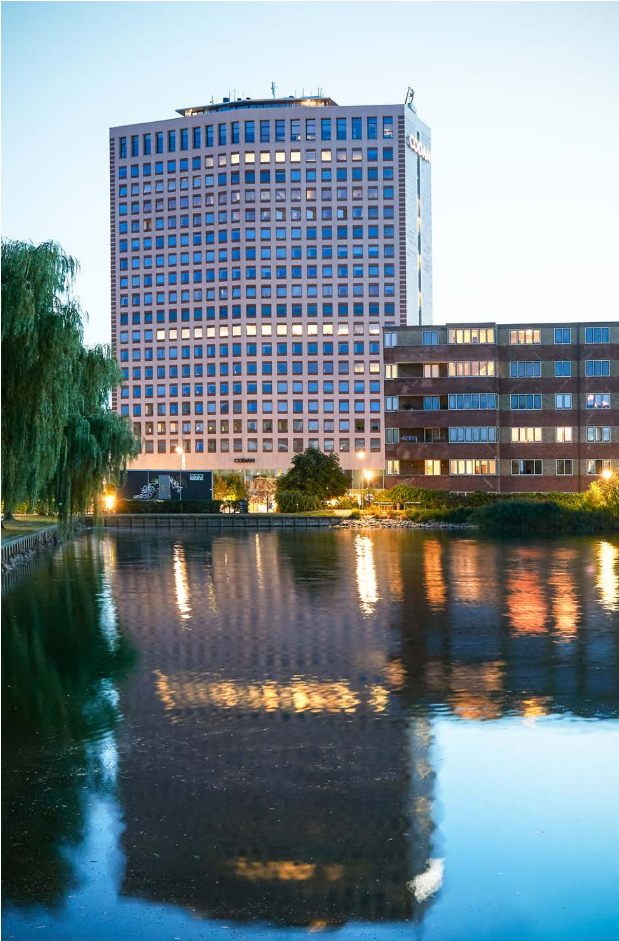
The Codan house in Copenhagen.
